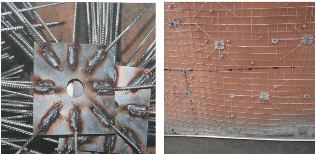
*Figures 7, 8: Strap with radial bars mounted on the anchor and the entire mesh before shotcrete process (photo auth.)*
