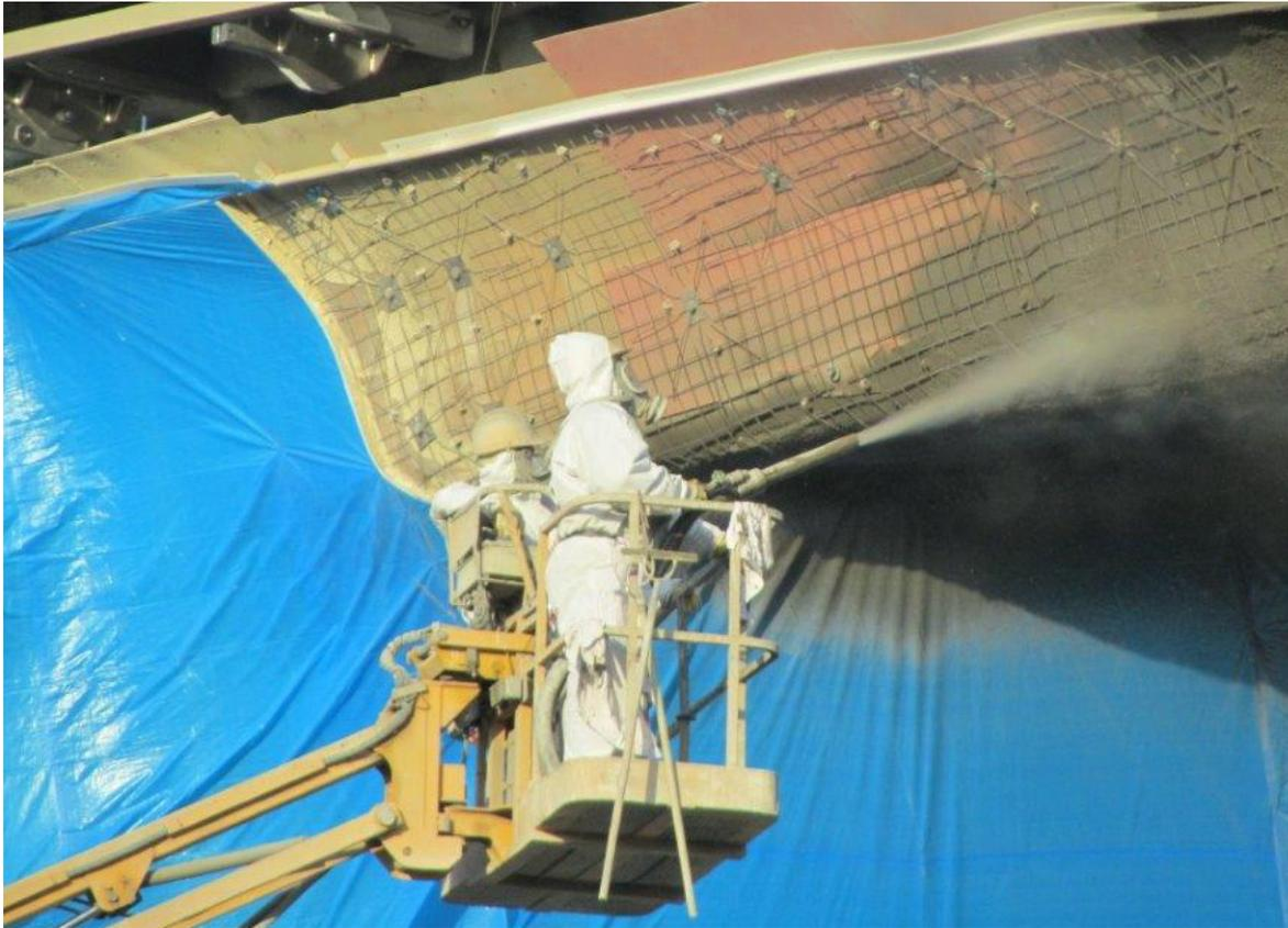
*Figure 10: Shotcreting process. In downing part ready shotcrete wall under the plastic foil which protected it against contamination by mortar blisters. The humid air upon foil cultivated young shotcrete and restricted shrinkage (photo auth.)*
