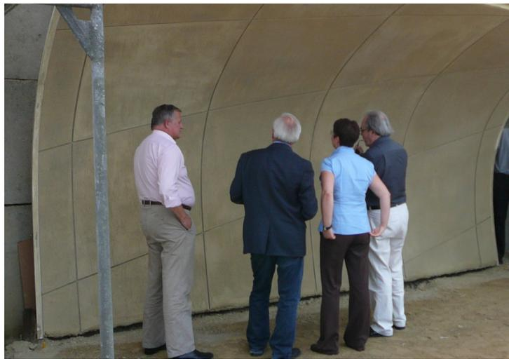
*Figure 5: Reference sample of curvilinear wall with the division into diamond-shaped elements at the contractor's polygon. Prof. Mahlamäki first from the right (photo auth.)*
