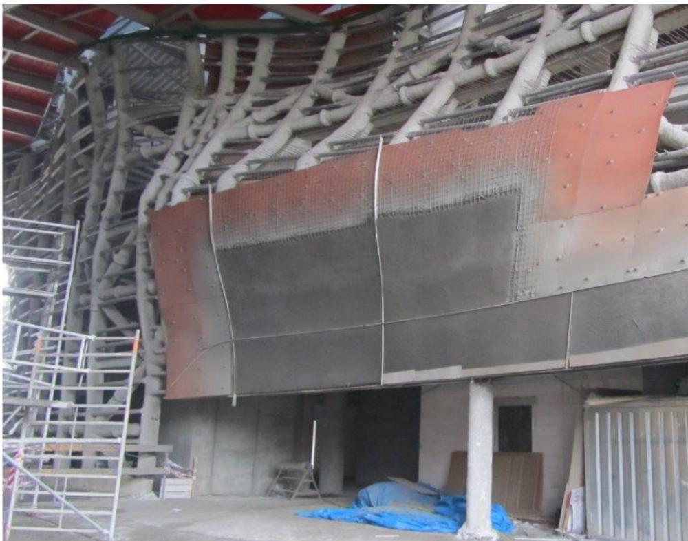
*Figure 9: Fire protected wall substructure, profiled special wooden plate as a stay-in-place formwork, anchors and reinforcement mesh, spacing strips, the first layer of shotcrete (photo auth.)*
