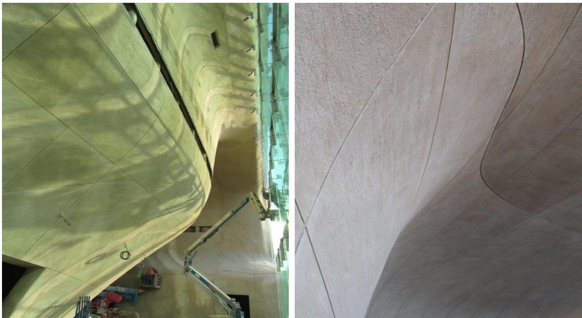
*Figure 11: Finished curvilinear walls; at the left wall with glazing (western exposure) (photo auth.)*
